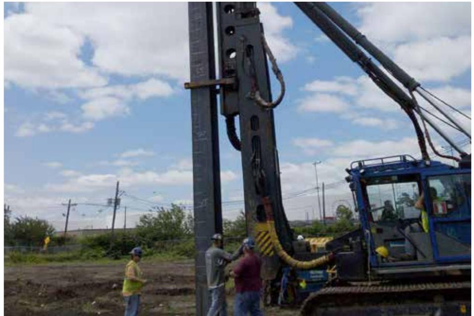
This project requires a driven pile foundation using HP 18 x 181 sections with pile tips driven to bedrock or stiff till, or drilled caissons to achieve the stiffness and load capacity specifications of the turbine manufacturers. A concrete pile cap of about 30 feet diameter at the tower base transfers the tower loads into the piles.
